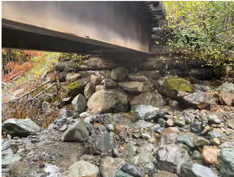
Right Bank Abutment when facing downstream
