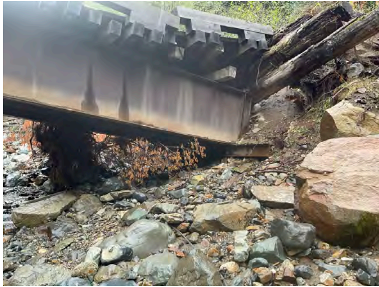
Left Bank Abutment when facing downstream
